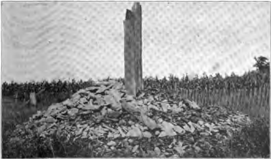
B.—Preparing a pile of limestone for burning. Note the alternate layers of coal and limestone.
